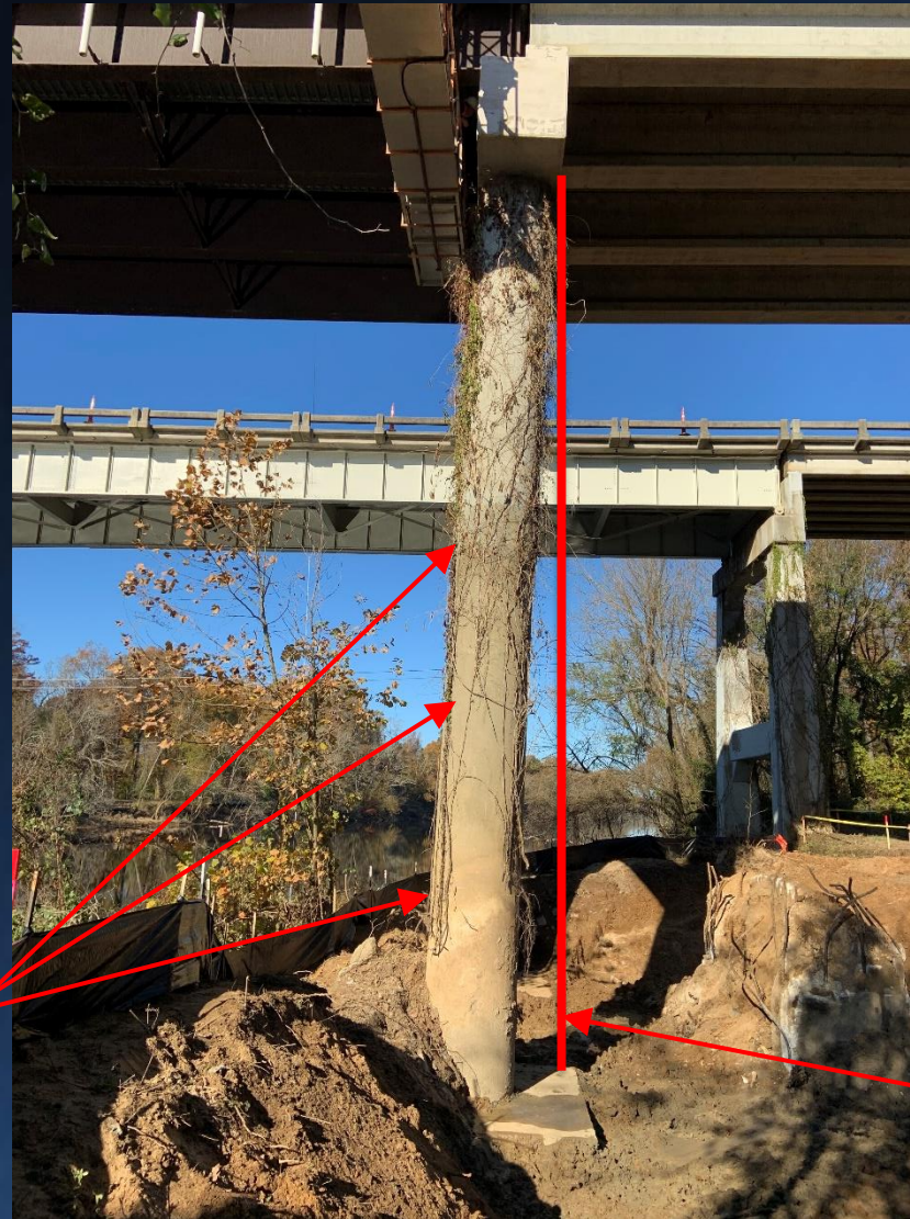
Tension Cracks on Both Columns
