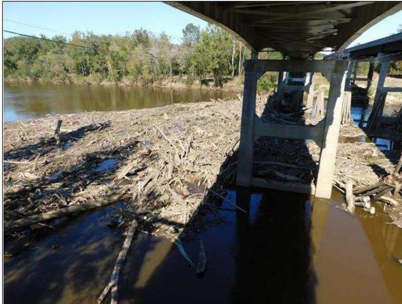
250' x 250' x 20' deep dirt and debris on upstream end of Spans 9-11 (PM)
